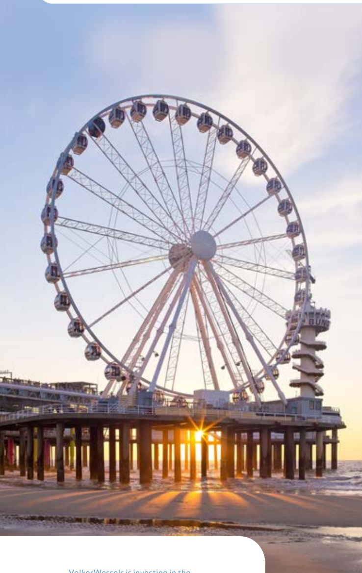
VolkerWessels is investing in the redevelopment of the pier at Scheveningen, which reopened in 2015.
