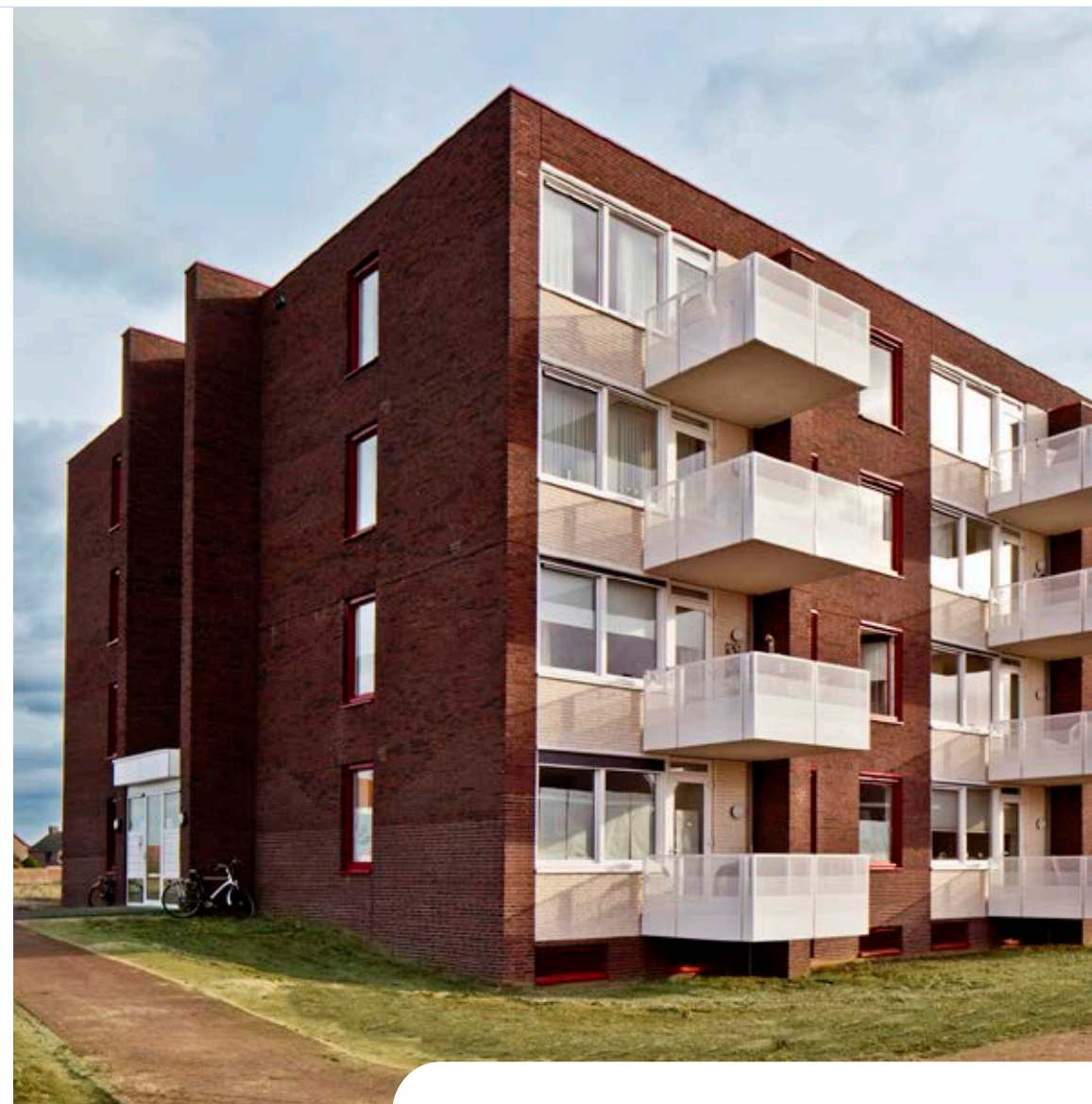
Oppe Brik project: a new residential area in Limburg province including 28 zero-energy bill apartments. The net-zero energy building is not connected to the gas main.
